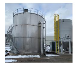
FRC's MBBR system uses floating biofilm media in aerated tanks to reduce BOD, nitrogen, and phosphorus with no need for RAS or MLSS monitoring.
