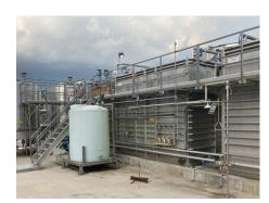
FRC biological wastewater treatment systems use MBBR and MBR technology to remove BOD, COD, and nutrients. Compact, efficient, and scalable solutions for industrial and municipal wastewater treatment.
