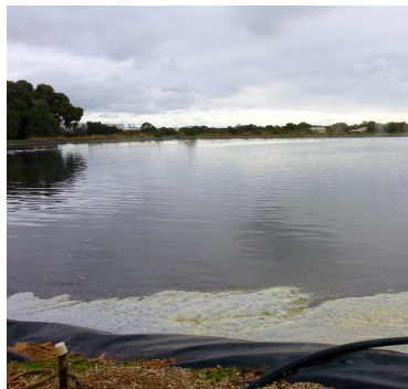
The lagoon system further reduces phosphorus and nitrogen concentrations.
